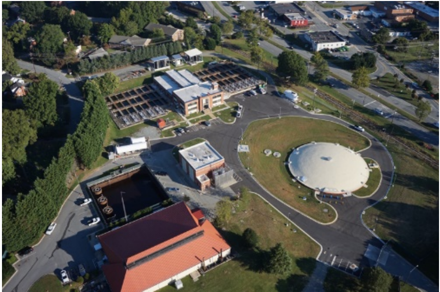
Mitchell Water Treatment Plant
