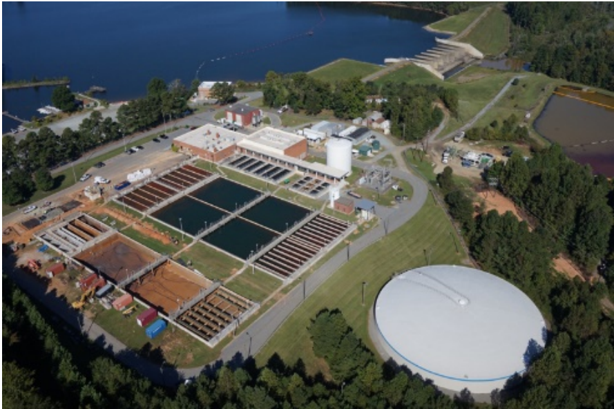
Lake Townsend Water Treatment Plant
